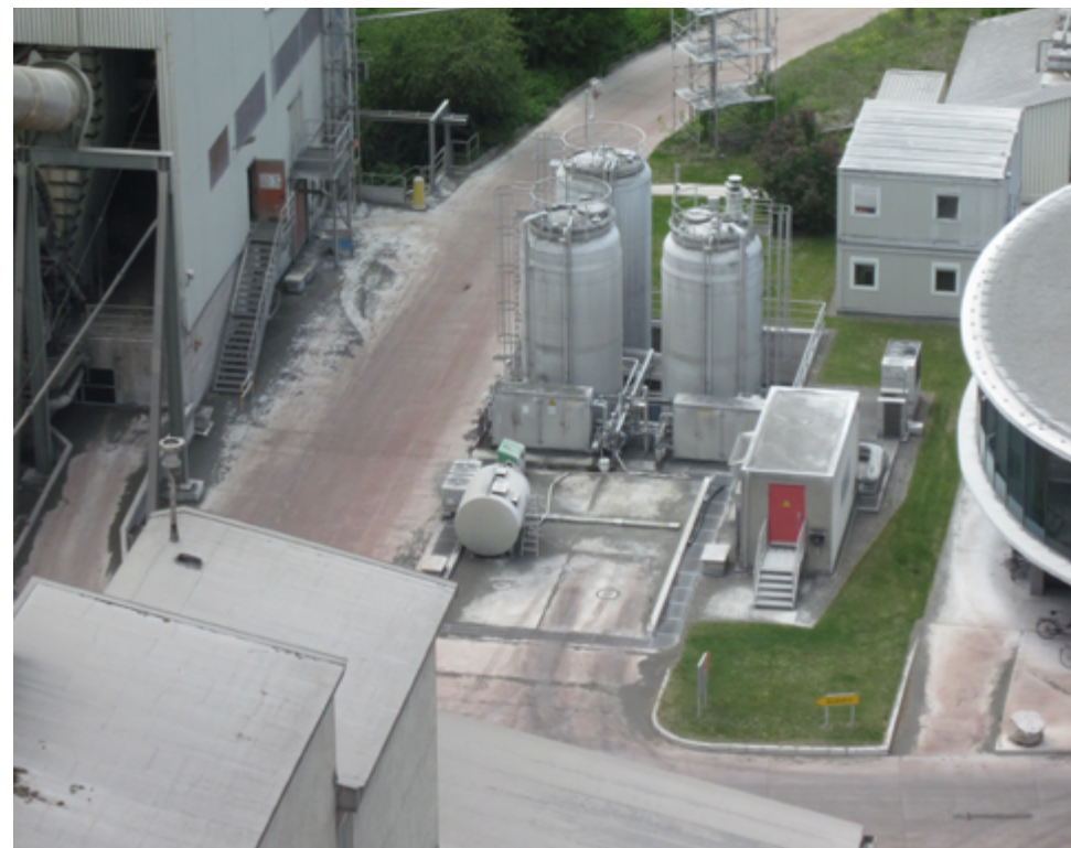
Picture 2: Flue gas agents (SNCR) tanks in Germany, 2012. (Source: MVW Lechtenberg & Partner).
