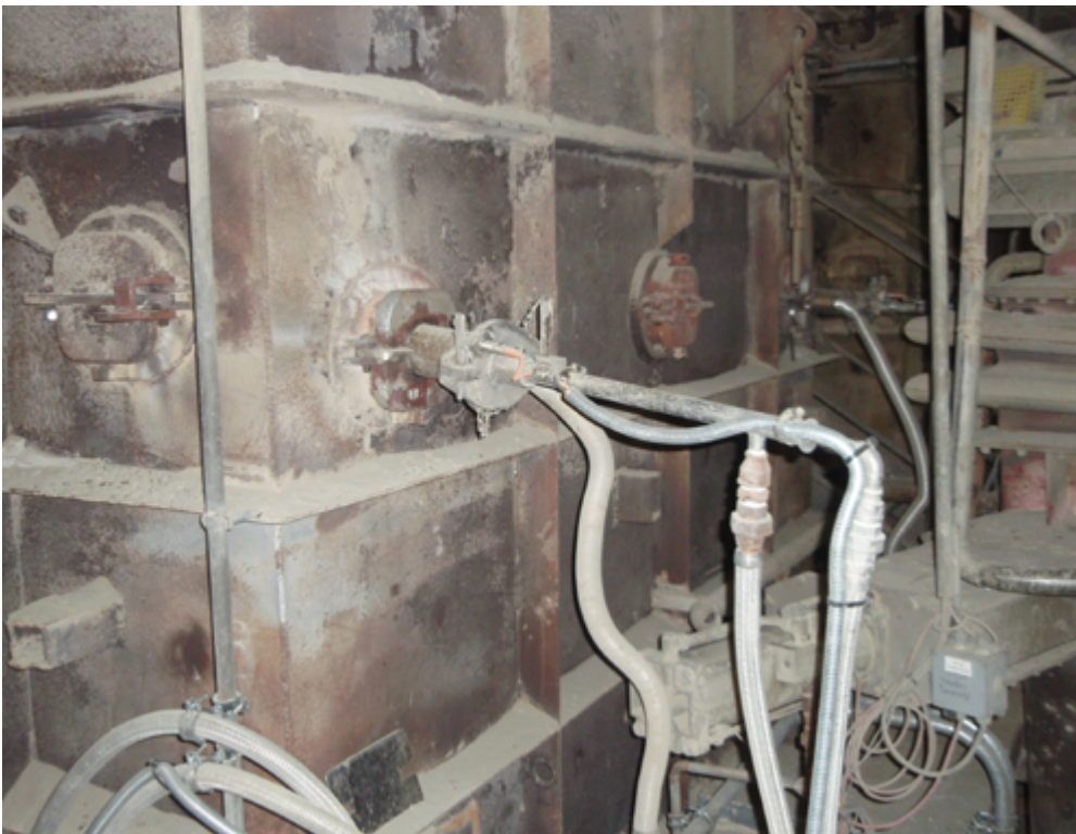
Picture 3: Gas probe kiln inlet. (Source: MVW Lechtenberg & Partner).
