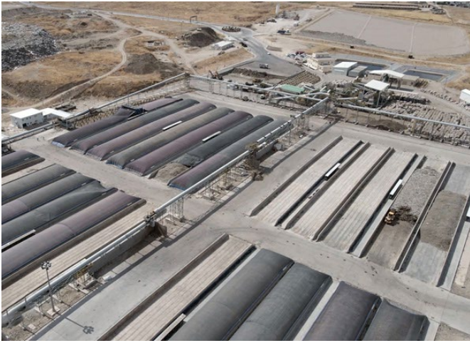
Figure 3: The Mechanical Biological Treatment facility of Faruk Investment Group in Sulaymaniyah, northern Iraq, is designed to take and process 480,000tpa of municipal solid waste (MSW) and generate 223,000tpa of RDF.
