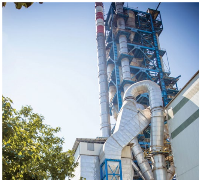
Figure 1: At the Lukavac plant, a five-stage cyclone preheater from KHD Humboldt Wedag and A TEC Production & Service calciner and bypass system were installed.
