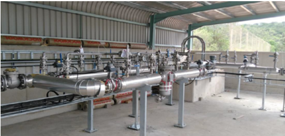
Figure 7: Pumping system for the tank. (Source: InterCement)
